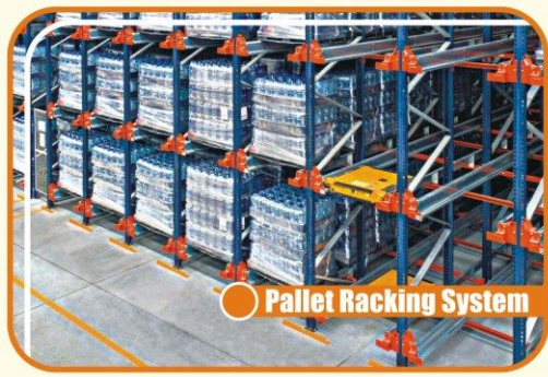
Pallet Racking System
